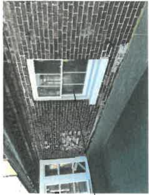
Window is same size as approved design but now a 3/3 rather than approved 6/6.
