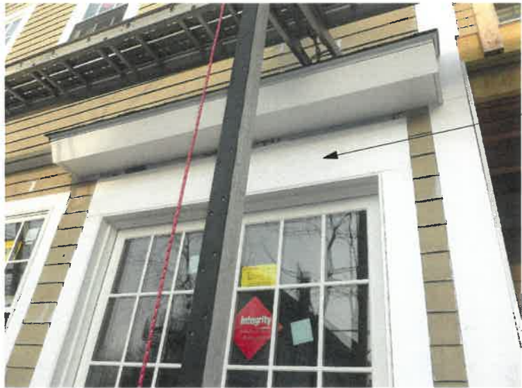
EXISTING REAR ROOF AND TRIM
