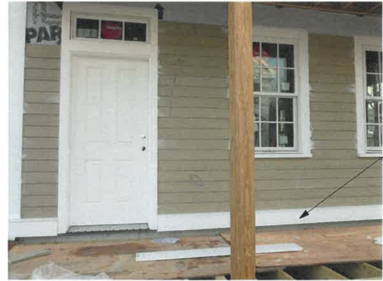
EXISTING FRONT PORCH AND TRIM
