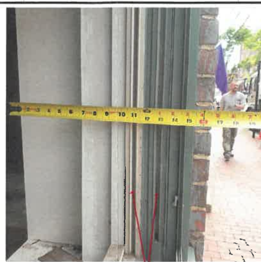
EXISTING WINDOW PHOTO 3
