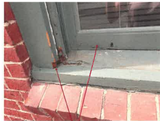
EXISTING WINDOW PHOTO 4
