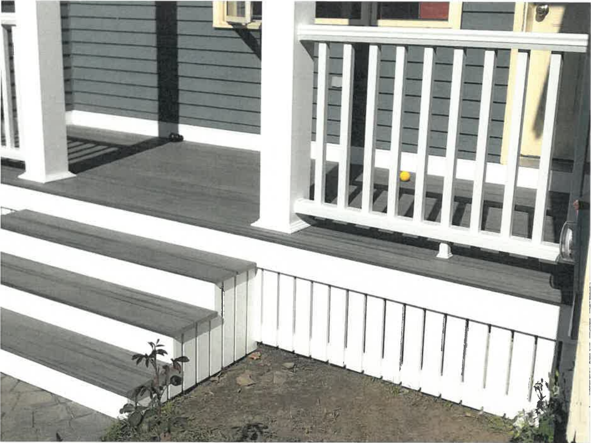
Photos of appearance of new deck, railings and trim from a similar project:
