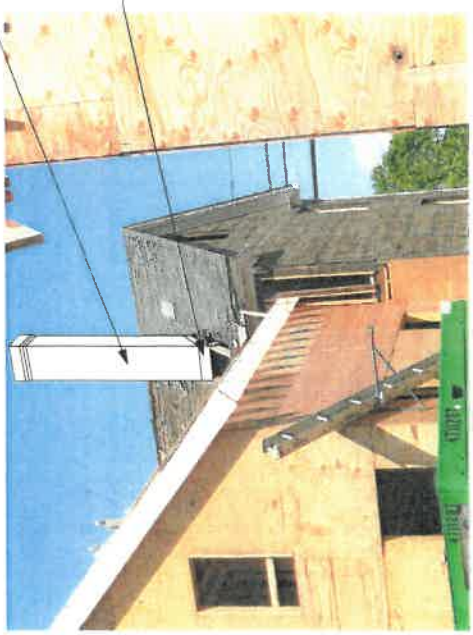
PROPOSED REBUILT FAUX CHIMNEY & LOCATION, MOVED OUT OF VALLEY TO PREVENT SNOW BUILDUP & WEATHER INFILTRATION PROPOSED METAL FLASHING TO PREVENT WEATHER INFILTRATION
