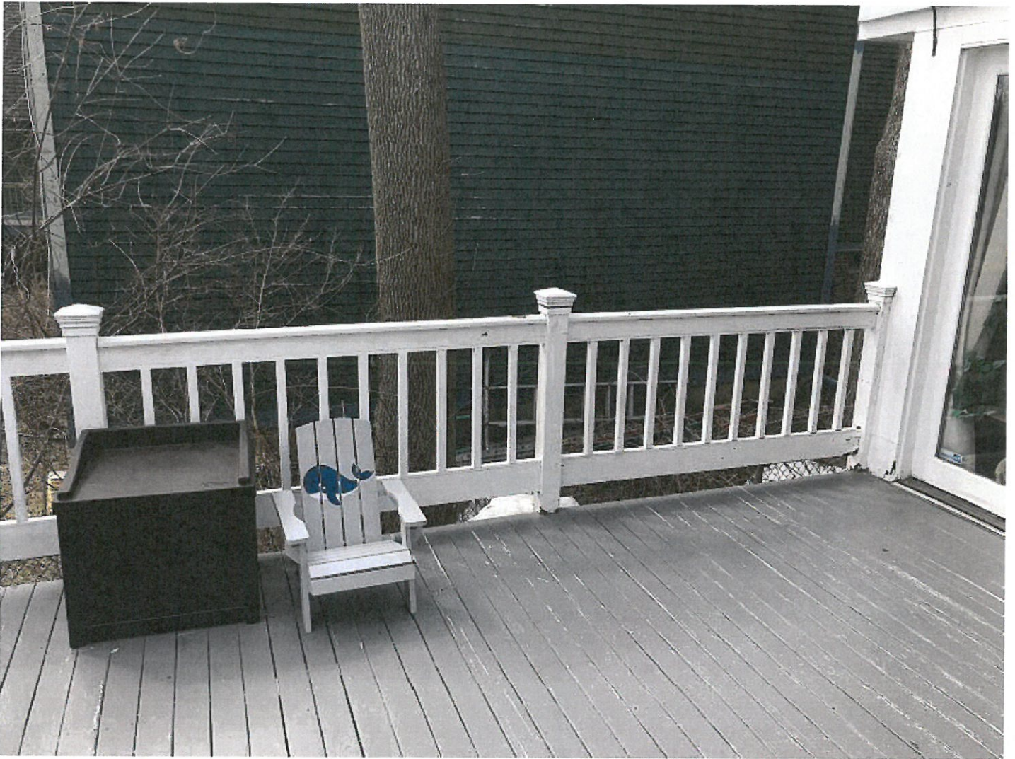
Existing Lower Deck
