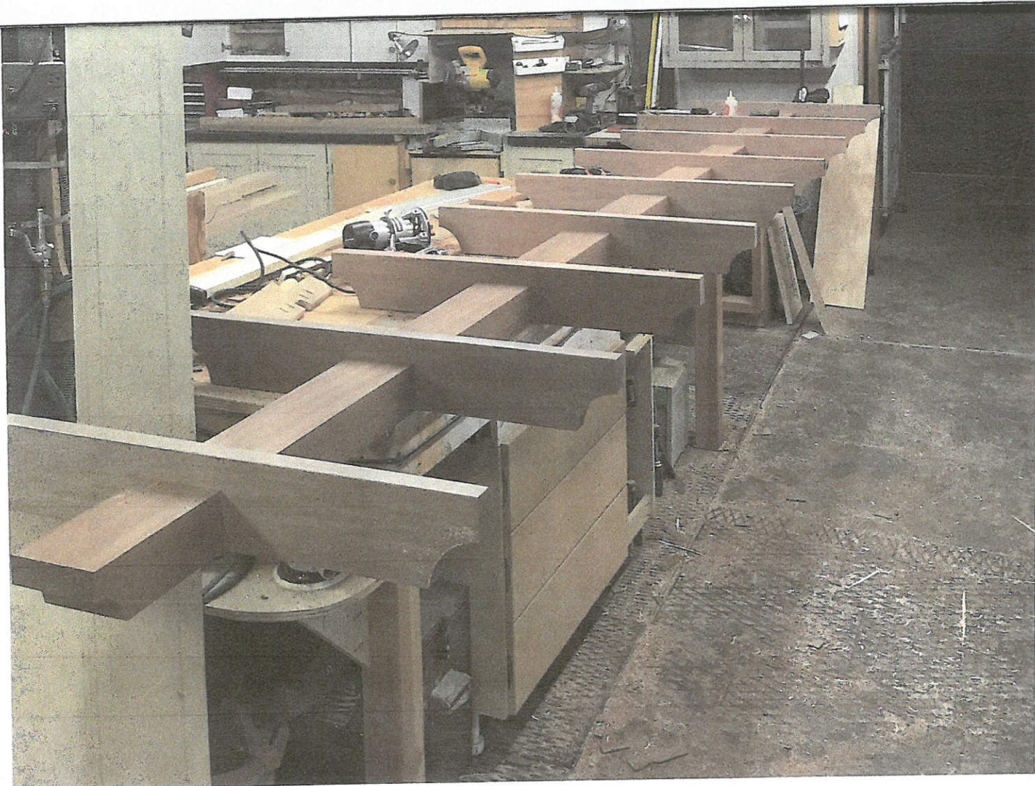
Pergola in Construction
