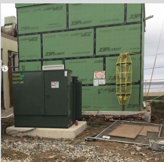
ELECTRICAL TRANSFORMER
