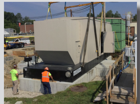
STANDBY ENGINE-GENERATOR
