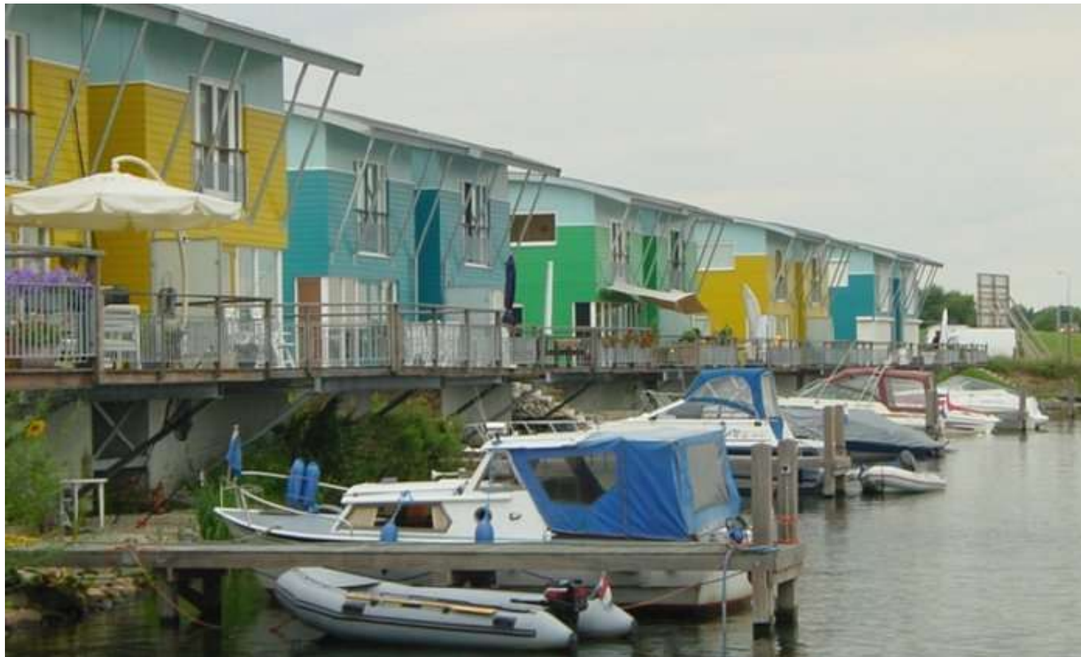
Amphibious housing in Maasbommel, Netherlands, can rise 18’.
