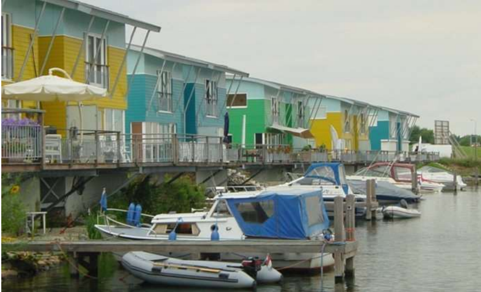
Amphibious housing in Maasbommel, Netherlands, can rise 18’.
