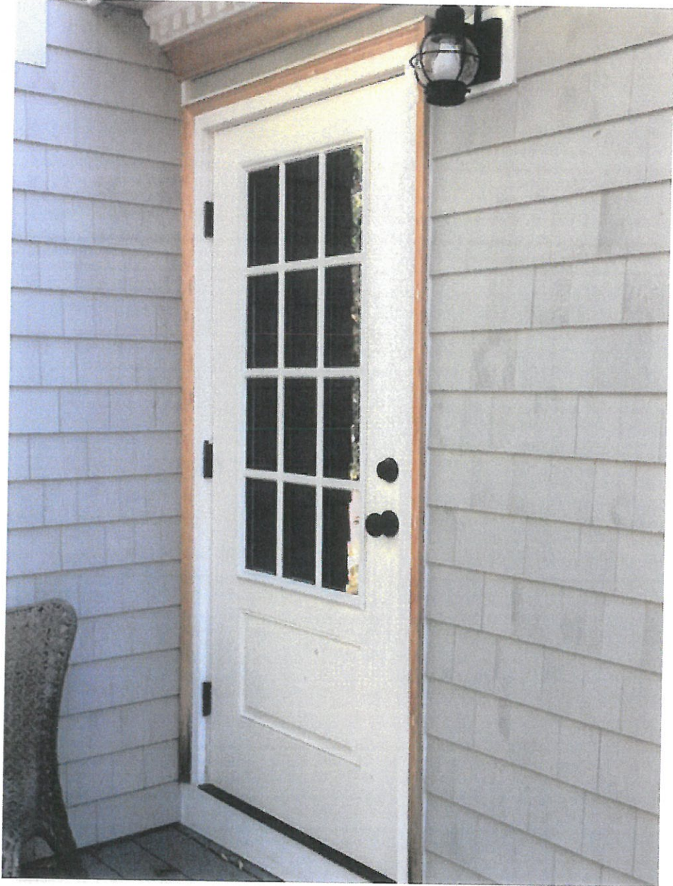
Picture #2 - New first floor door. New Basement Door to Match.
