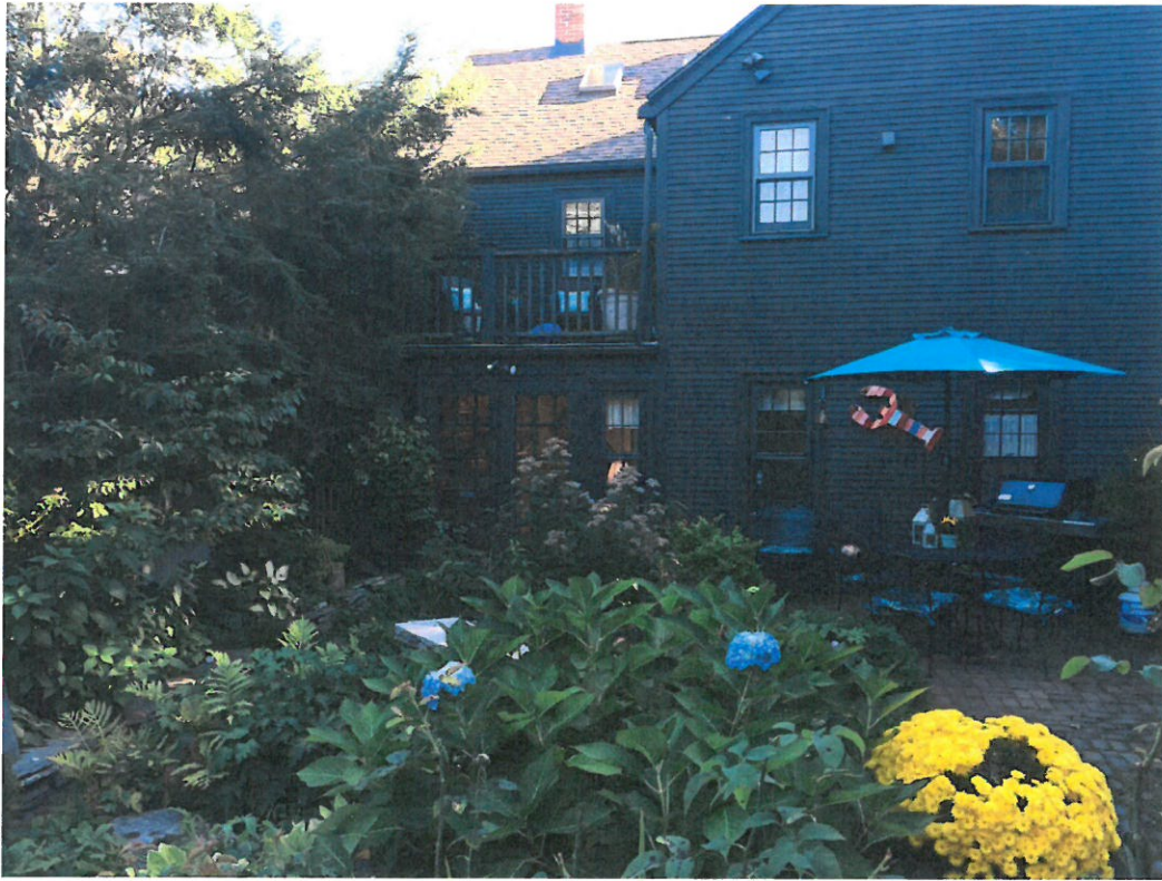
17 Hunking – Existing French doors
