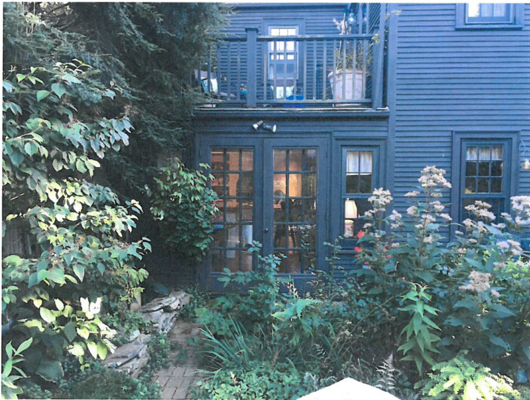
17 Hunking – Existing French doors
