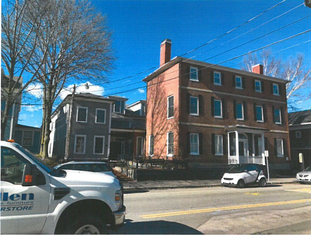
Photograph 2 – slightly South from photograph 1, also directly across the street from 133 Islington street.
