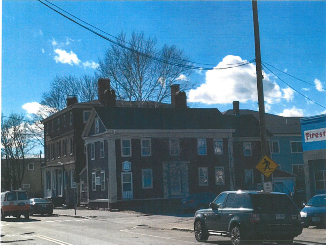
Photograph 4 – This taken from further Northwards along Islington street, facing west.
