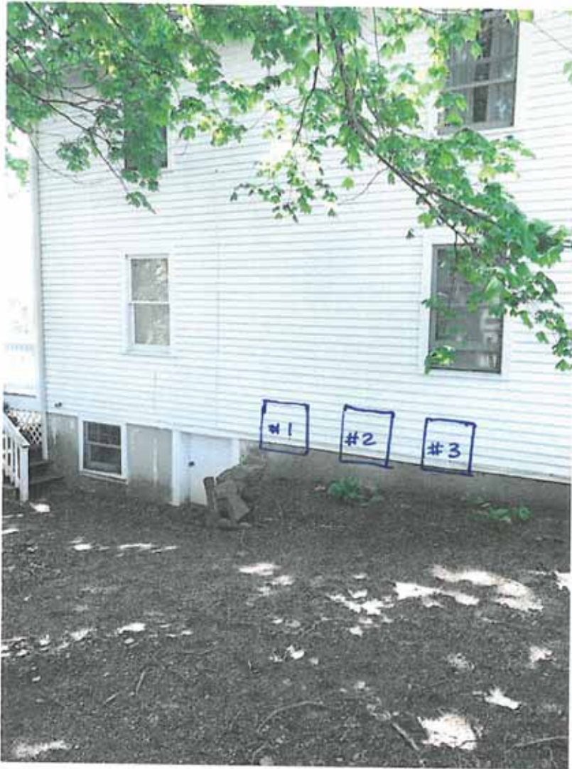
Eastern Side Rear – Basement Access
