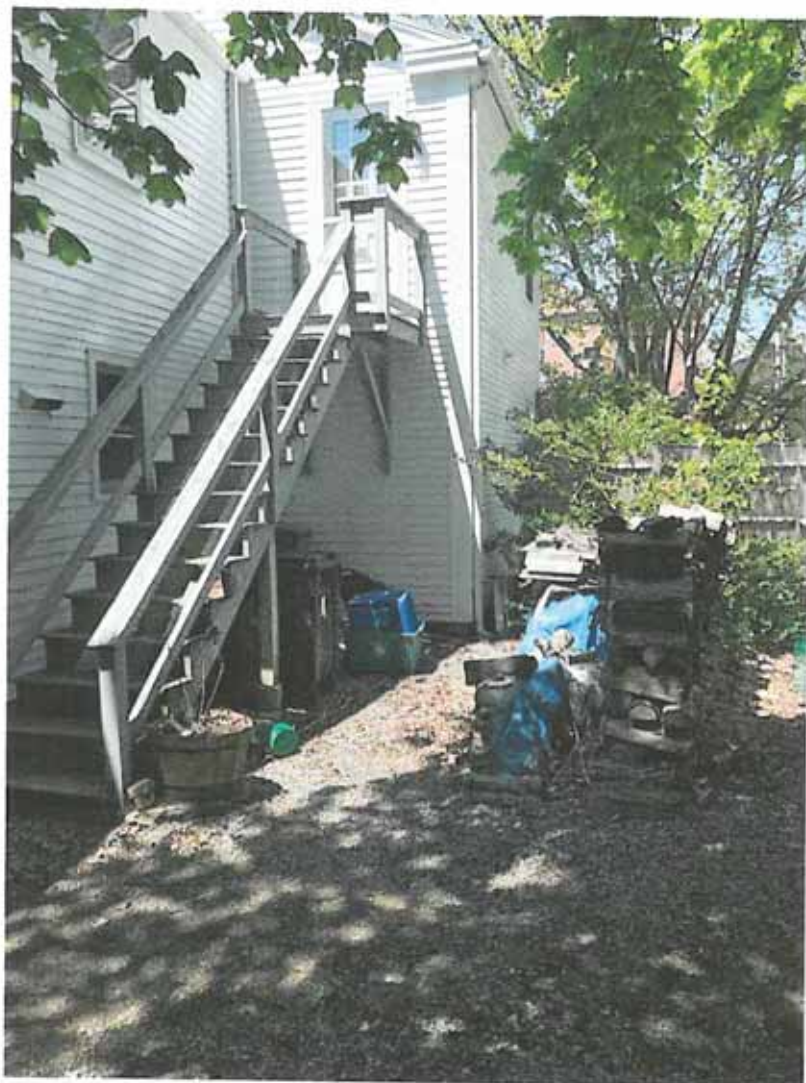
Exterior Staircase on Eastern Side
