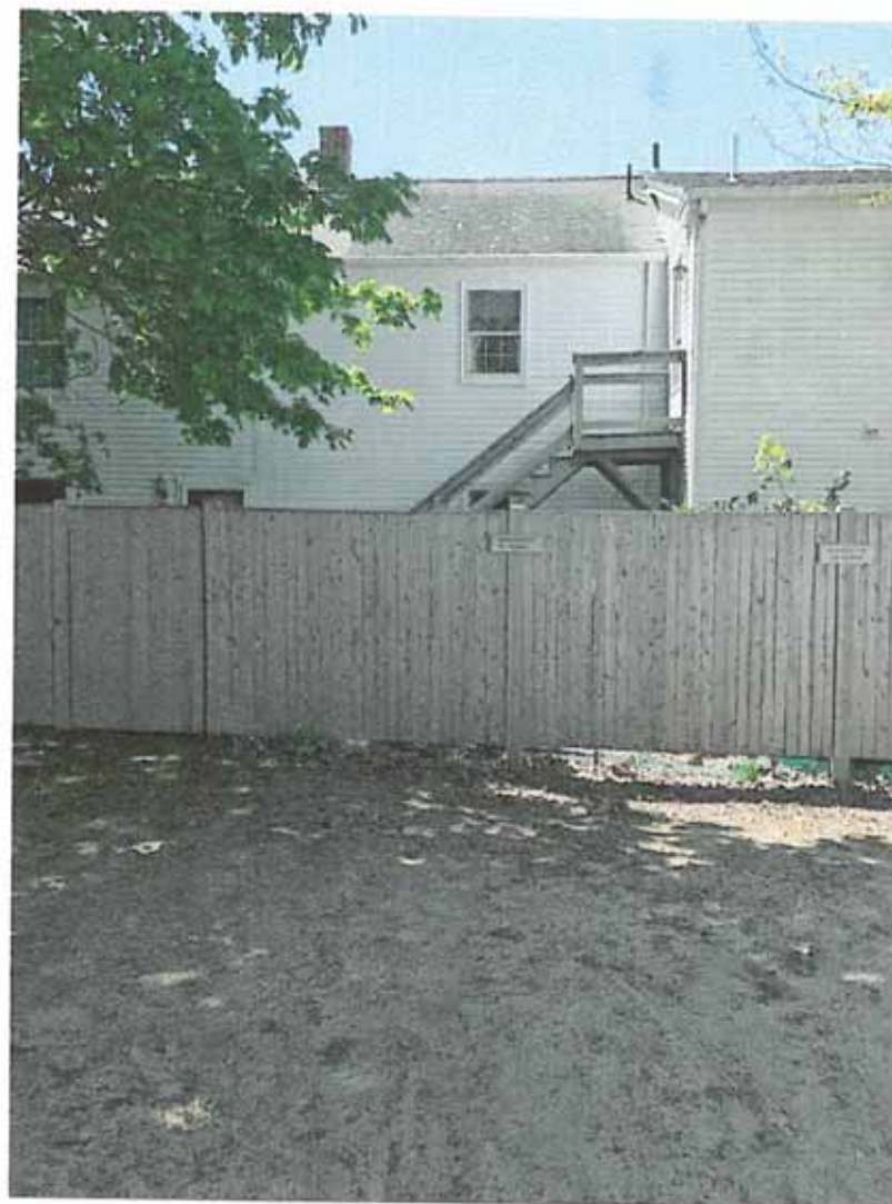
Exterior Staircase from Parking Lot
