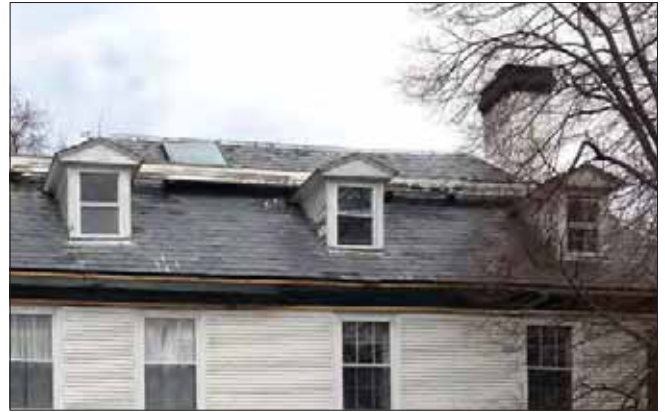
The roof surface, balustrade and cornice were damaged by heavy snow and were replaced to match the historic conditions. (Refer to photograph below.)
