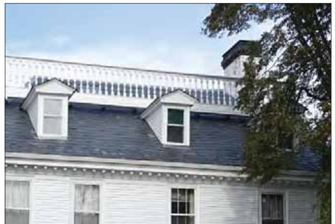
The roof, balustrade and cornice were replaced using compatible materials, that convey an appearance that is similar to the historic condition prior to storm damage.
