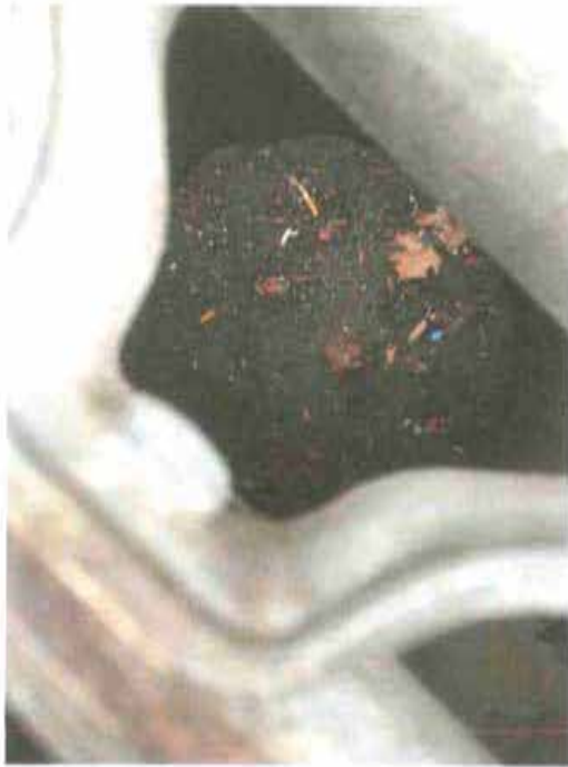
This is the gutter outside NJM Gallery all of this is flowing into the town water and contaminating it.
